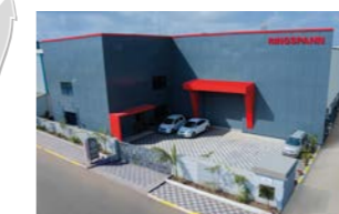
RINGSPANN Power Transmission India Pvt. Ltd., Inde
